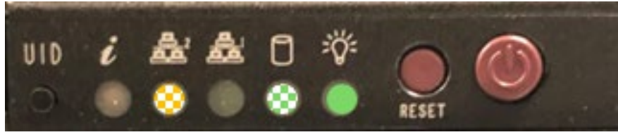
Figure 20: Server when switched ON. Yellow and green patterns indicate flashing
